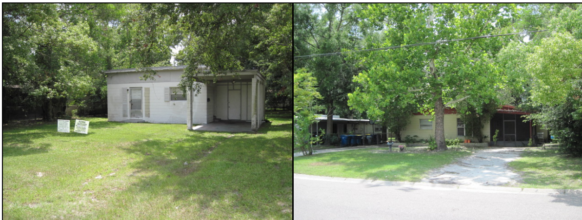
Single-family homes to be demolished along Wake Forest Avenue.
