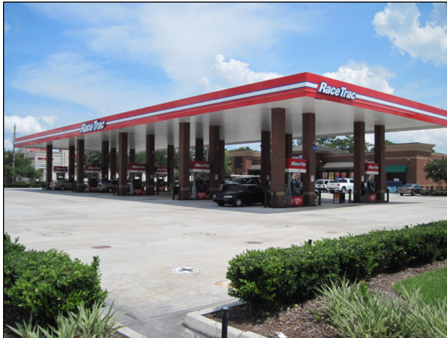
RaceTrac gas station east of the property (PUD 2008-552-E).
