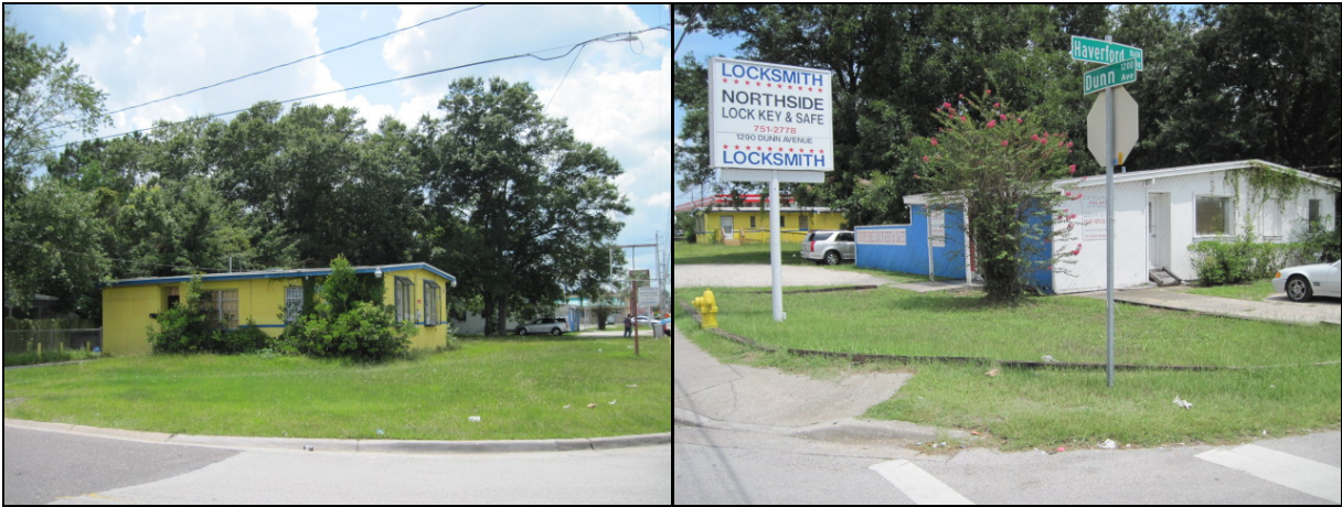
Single-family homes to be demolished along Dunn Avenue, between Wake Forest Avenue and Haverford Road.
