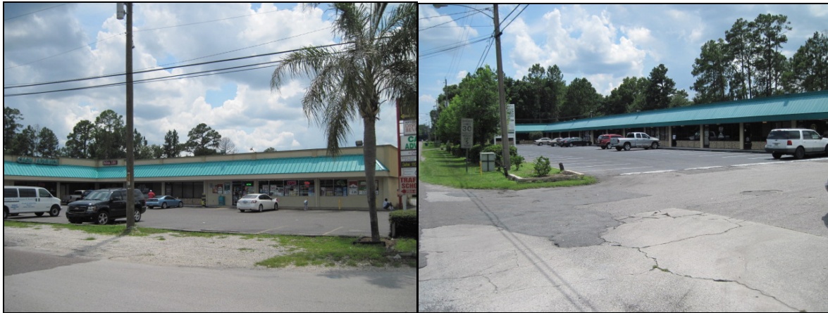
Commercial Shopping Center to the West across Haverford Road.
